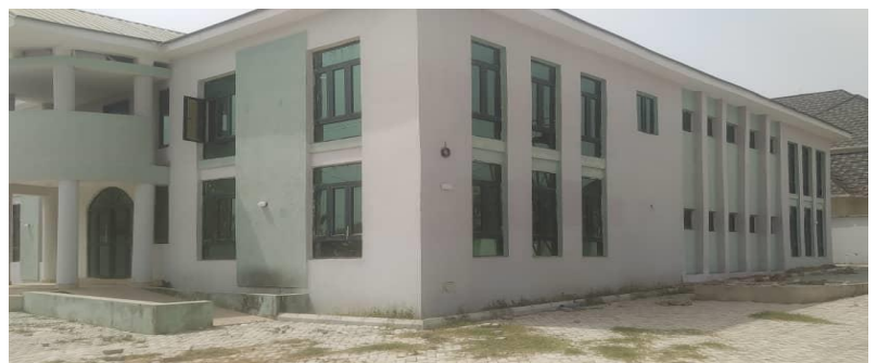
Side view of Benue State Office complex
