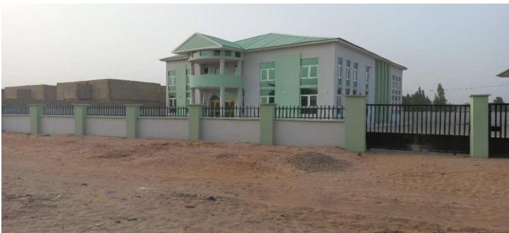
Katsina State Office: Completed
