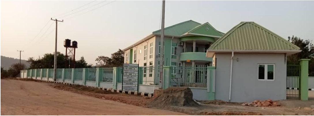
Ekiti Prototype Office Completed
